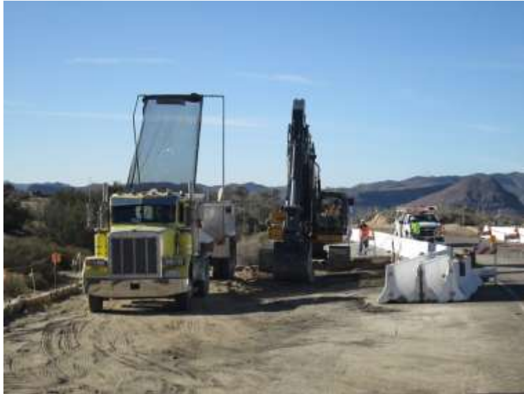
Photo 1: Trucks transporting bulk materials covered in accordance with MM AQ-1.
